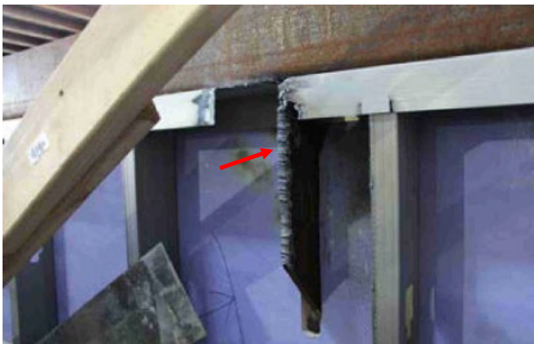
Figure 3. Trimmed knife plate edge (indicated).
