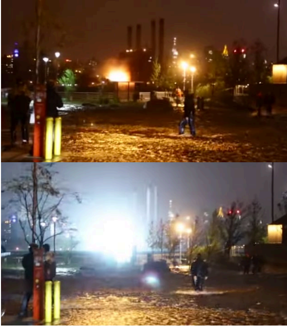
Figure 12. Sequence of still images from a video published on YouTube of an apparent arcing and explosion event at the East River Complex during Sandy.
